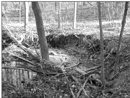
Severe erosion in a headwaters tributary of the Occoquan Reservoir.
