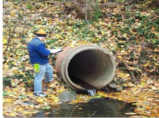
Visual inspections are used to look for any signs of flow discharges in storm drain manholes or outfalls. If found, samples are taken to measure flow, color, odor, oils, floatables and water quality parameters.
