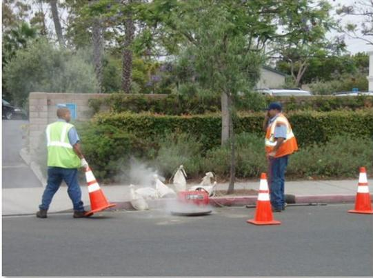
Smoke is introduced into the sewer to see where it surfaces to find the source of the discharge.
