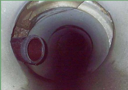
5. Sewer lateral directly connected to the storm drain system.
