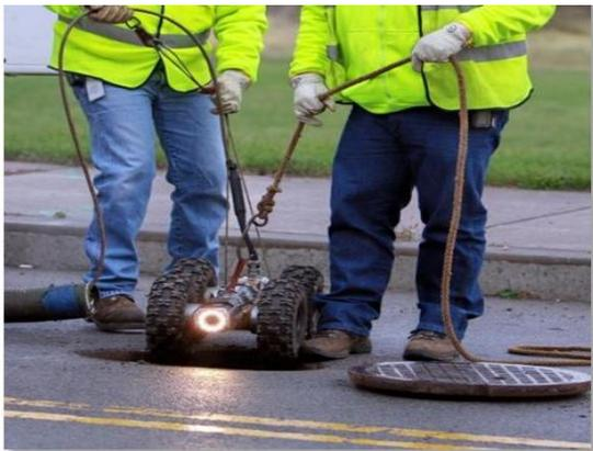
A remote video camera assesses the condition of a storm or sewer pipe to look for discharges.
