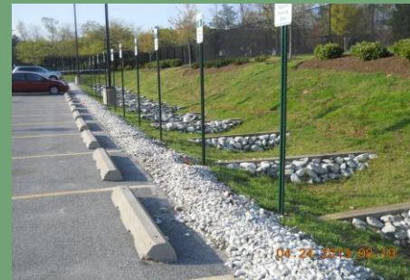
Example of a water quality swale at the edge of a parking lot
