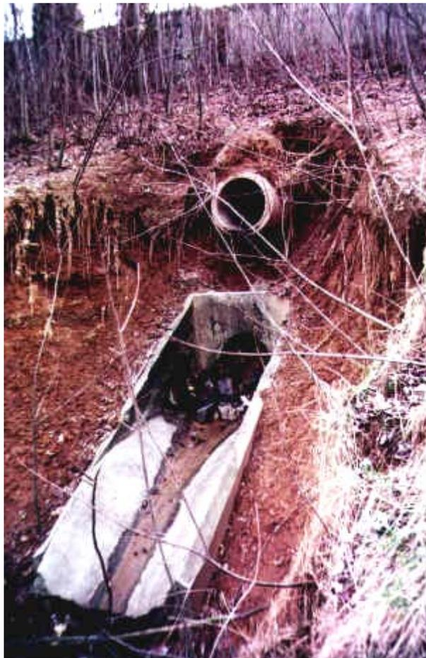
**Figure 6- Stormwater Impacts Resulting in Severe Channel Degradation**
