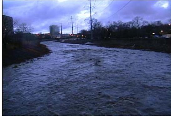
When the channelization project of Four Mile Run was conceived in the 1960's, the sole objective of the project was flood protection and, to that end, the project has been a success; no floods have occurred along the 2.3 mile channel since its construction. Although successful in flood control, with respect to aesthetic and environmental attributes the channeled section of Four Mile Run leaves much to be desired.
