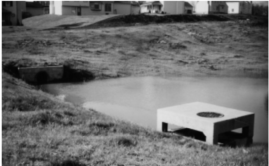
FIGURE 1.2 Typical Structural BMP – Wet Pond
